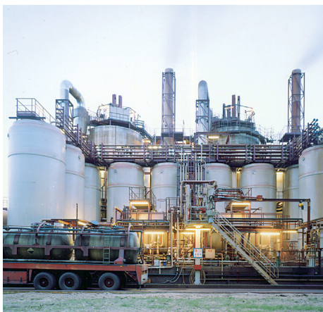
Fig 5 Acid regeneration plant with zero emission discharge
